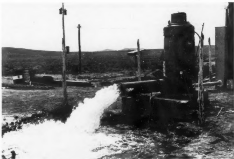
DEEP WELL TURBINE pump discharges 3,500 gallons per minute from drill hole which taps fissure at 500 foot depth. Electric power was brought to the mine site to drive the 440-horsepower Fairbanks-Morse pump. DeWatering of vein precedes sinking.
